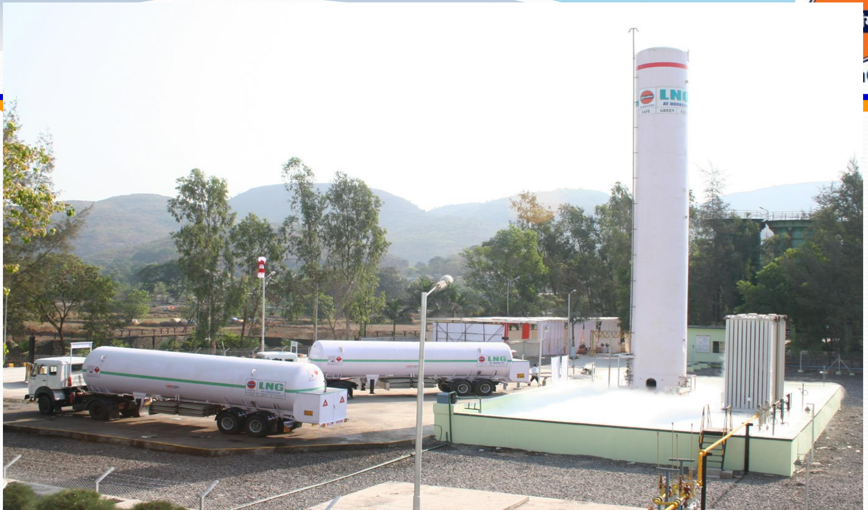
LNG Storage & Regasification facility at M/s H &R Johnson Ltd
