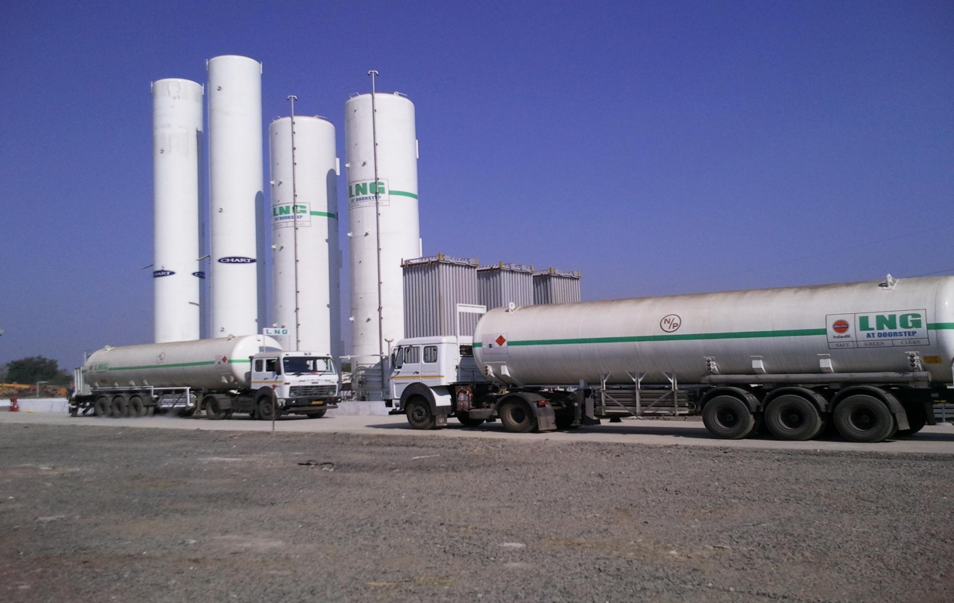
LNG Storage & Regasification facility at M/s Hindustan National Glass Ltd., Nasik
