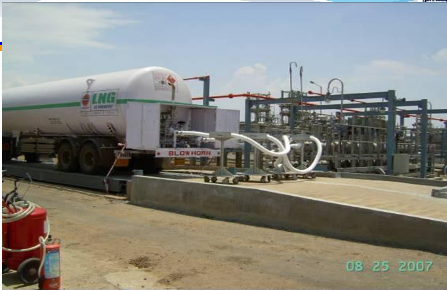
Tanker loading facilities at PLL, Dahej
